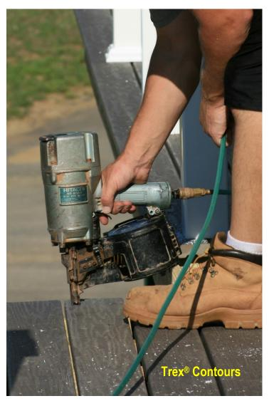
Ballistic NailScrews® (BNS) are collated screws that install with a pneumatic nailer. Using them can increase productivity, lower labor costs, provide high quality and durability to your work, and reduce the operation stress associated with other collated screw systems.
