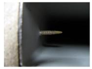
For the best pull-out resistance, only allow three to five threads of the NailScrew® through the metal substrate.
